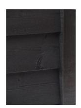
Fine sawn finish with one stain resistant primer coat and one top coat of black paint.
